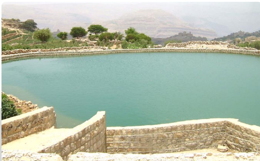
SFD-supported rainwater harvesting projects give communities sustainable sources of water (Al-Sawdah, Amran)
